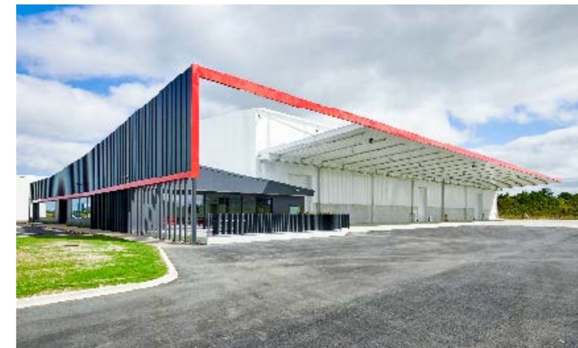
New distribution center with office building • New Zealand
